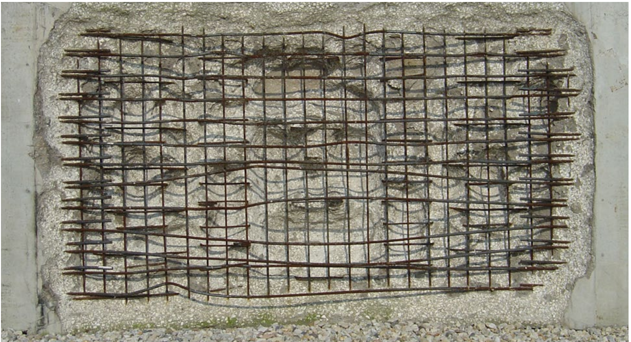
If the concrete is heated quickly and high thermal stresses occur, considerable damage may be caused to the concrete structural elements.
